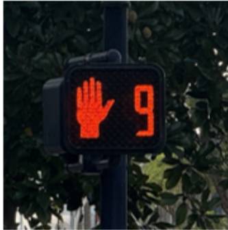
Pedestrian Countdown Signals provide pedestrians with a clear indication of how many seconds remain to safely cross.
