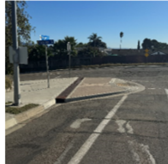
Curb Pop Outs or Curb Extensions shorten pedestrian crossing distances and serve as a traffic calming mechanism.
