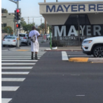
Advance Stop Bars/Limit Lines direct drivers where to stop at intersections and mid-block crossing locations, providing separation between the vehicle and crossing pedestrians.
