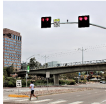
Pedestrian Hybrid Beacons are traffic control signals that help pedestrians and bicyclists cross mid-block across high traffic roadways.
